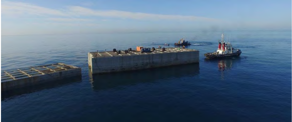
Diagram 3-8: Caisson control platform and equipment to position and sink them.
